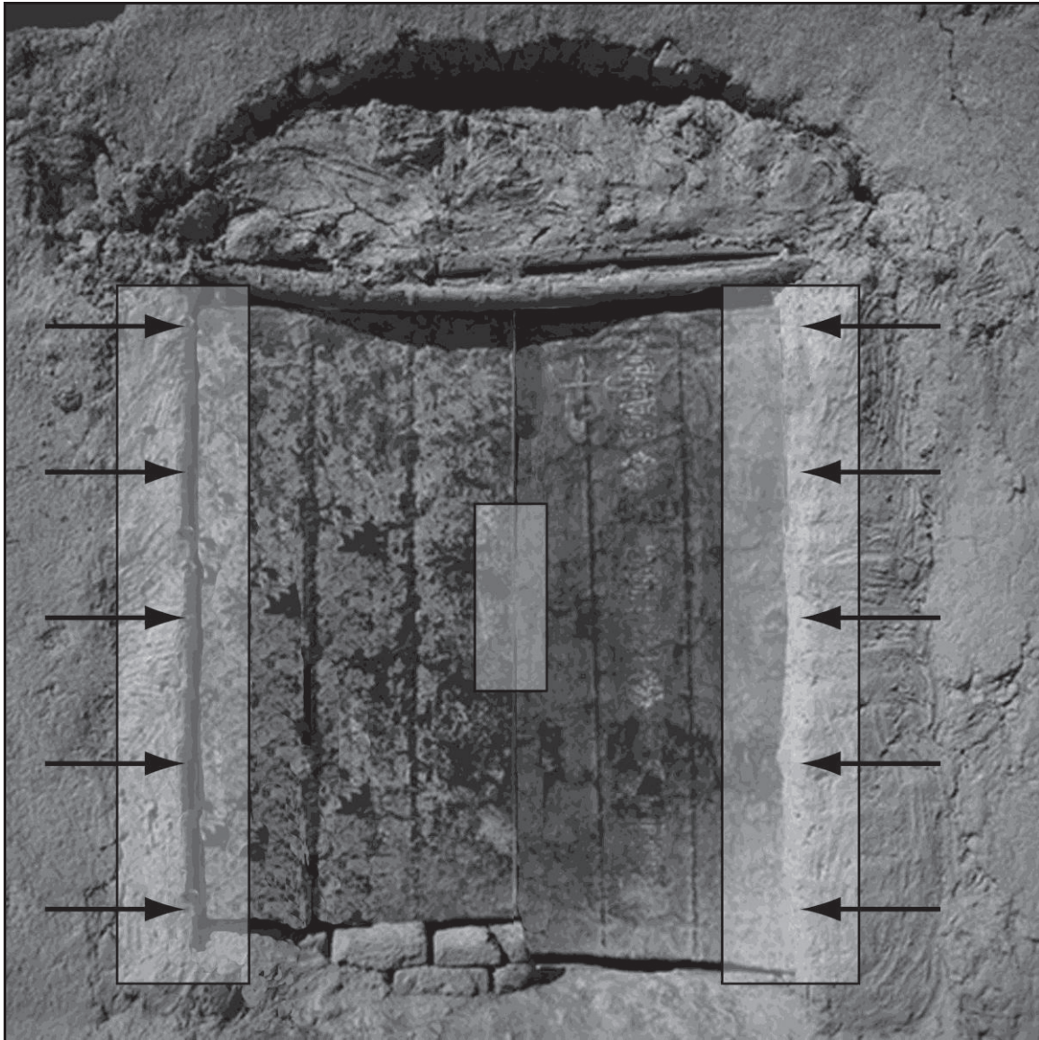
Figure 5-7. Steel door with clay frame breaching points
