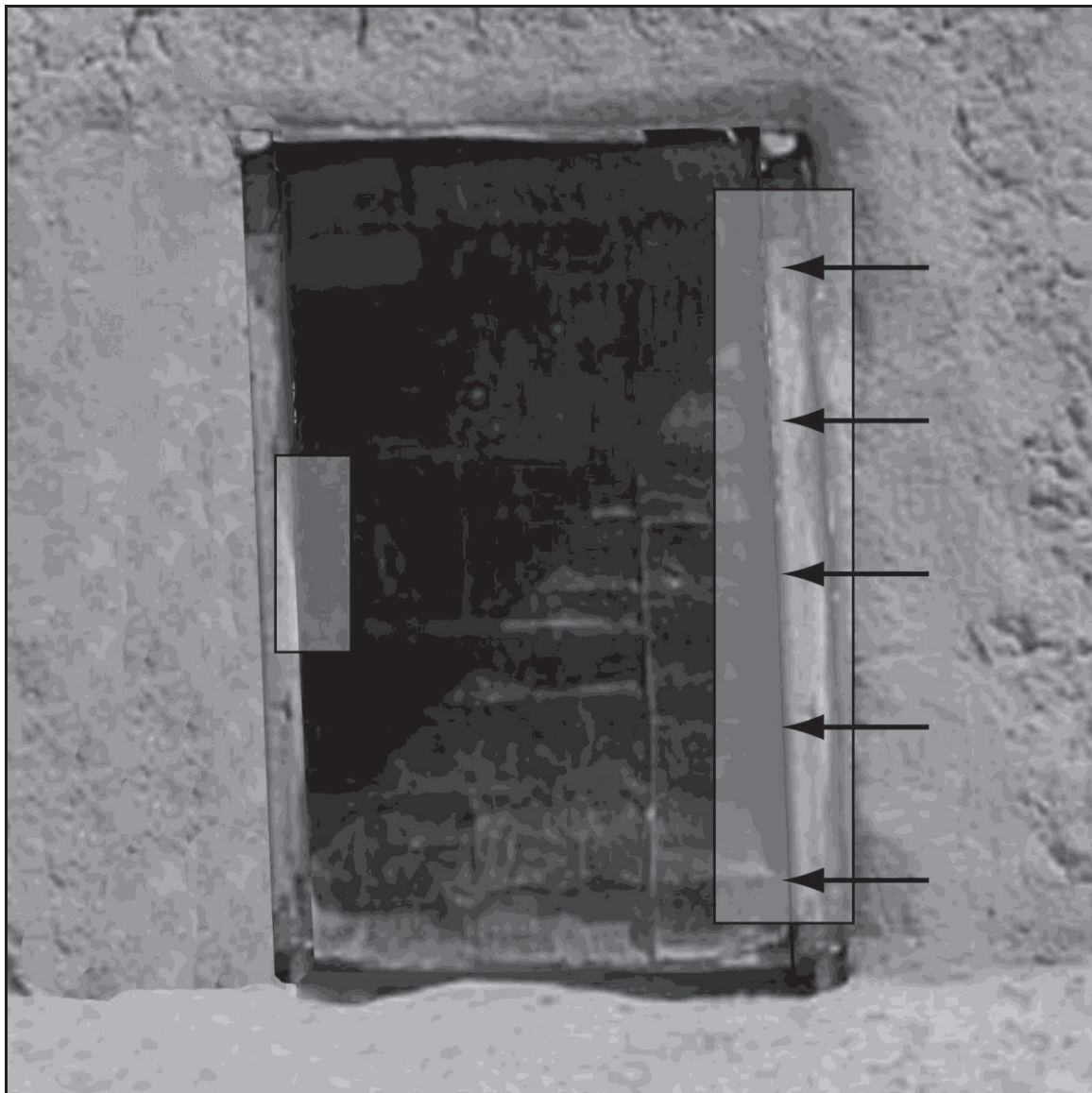
Figure 5-6. Steel door with wood frame
